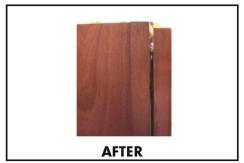
If the door does not appear to be parallel to the cabinet frame it can be easily corrected by using the Salice auto-adjustment depth screw. Simply adjust the top hinge inward and the bottom hinge outward
